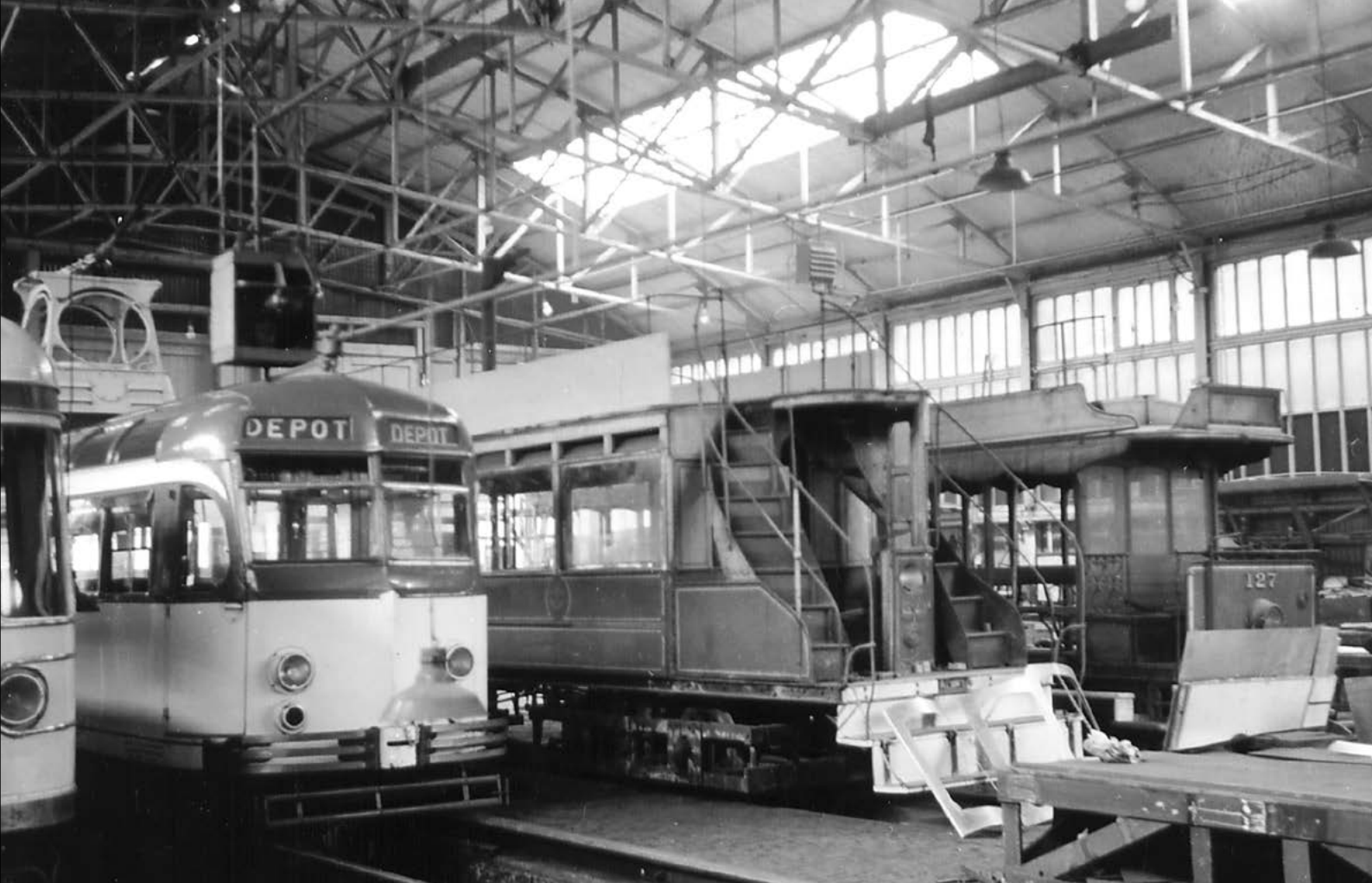
An interesting scene in the old Body Shop in 1960, showing Vambac Railcoach 208 with Dreadnought 59 and Crossbench 2 both being restored for the Anniversary in September. The structure of the building identifies it as originally having being an aircraft hangar. (Author)
