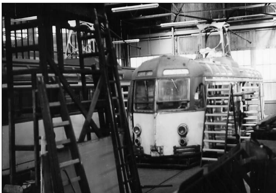
Inside the Body Shop in April 1964, showing two Brush cars 286 and 294 being repanelled and having their sliding sunshine roofs removed. (Author)
