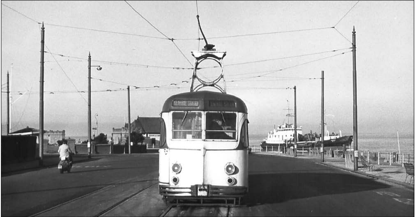
A maritime view of 270 at the Ferry with the dredger sailing in, and the lifeboat house behind the tram. (Author)
