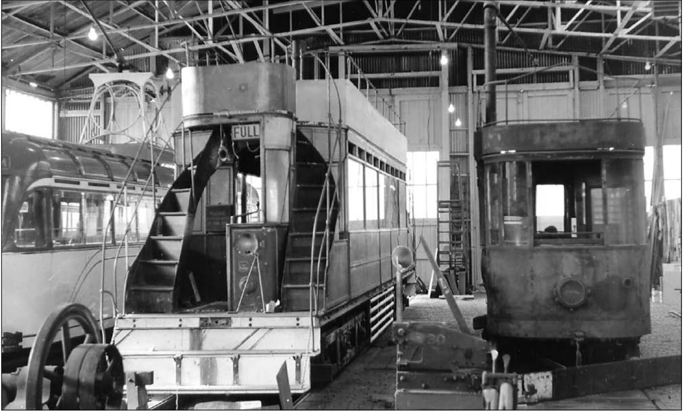
A fascinating scene in the Body Shop with Dreadnought 59 newly fitted with folding steps and upper-deck panels, joined by ex-conduit car 4 still fitted with the snowplough in February 1960. (Author)
