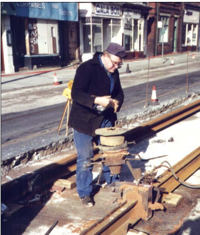
Views of welding track in North Albert Street, Fleetwood in February 1990, showing first fitting the crucible over the clamped rail-joint, and then the burning magnesium filling the rail-joint. This is how the rail-joints were welded on the Marton route in 1949. (Author)
