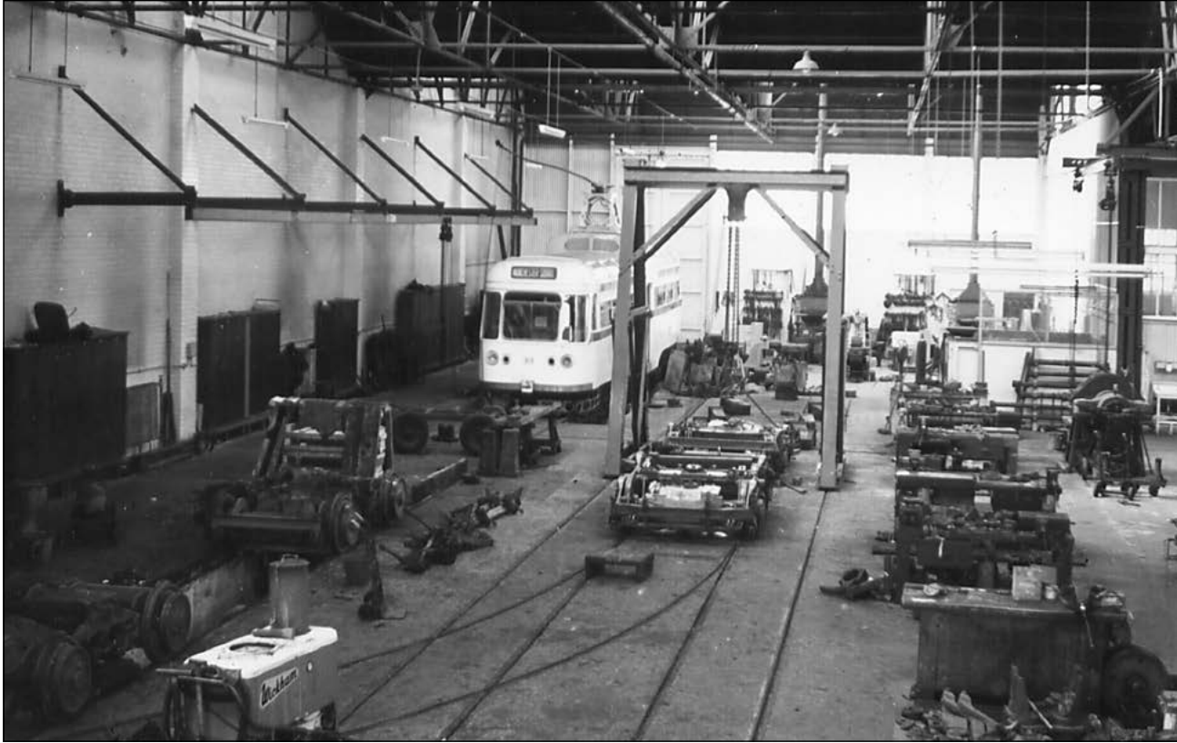
The new Fitting Shop in April 1964, showing Coronation 319 standing over the wheel drop pit. A pair of M & T bogies are nearby, and under the lifting frame a pair of EE bogies can be seen. (Author)
