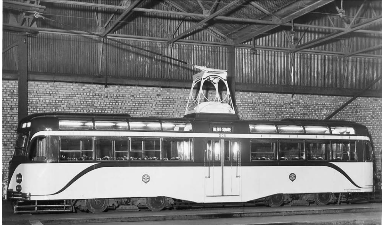
A profile of 208 with Maley & Taunton bogies fitted with track brakes. Inside the tower is the Vambac equipment in a cream dome, whilst the saloon boasts the fluorescent lights. (Author's Collection)
