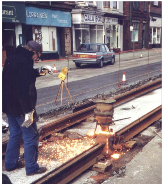
Views of welding track in North Albert Street, Fleetwood in February 1990, showing first fitting the crucible over the clamped rail-joint, and then the burning magnesium filling the rail-joint. This is how the rail-joints were welded on the Marton route in 1949. (Author)
