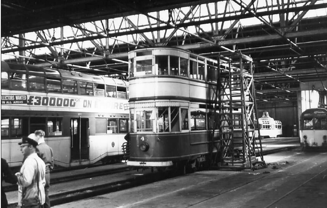
In August 1964, Standard 48 is being prepared for it to leave for Portland, USA, and the crews wait to take out other cars, possibly Balloon 247 (710) nearby. (Author)
