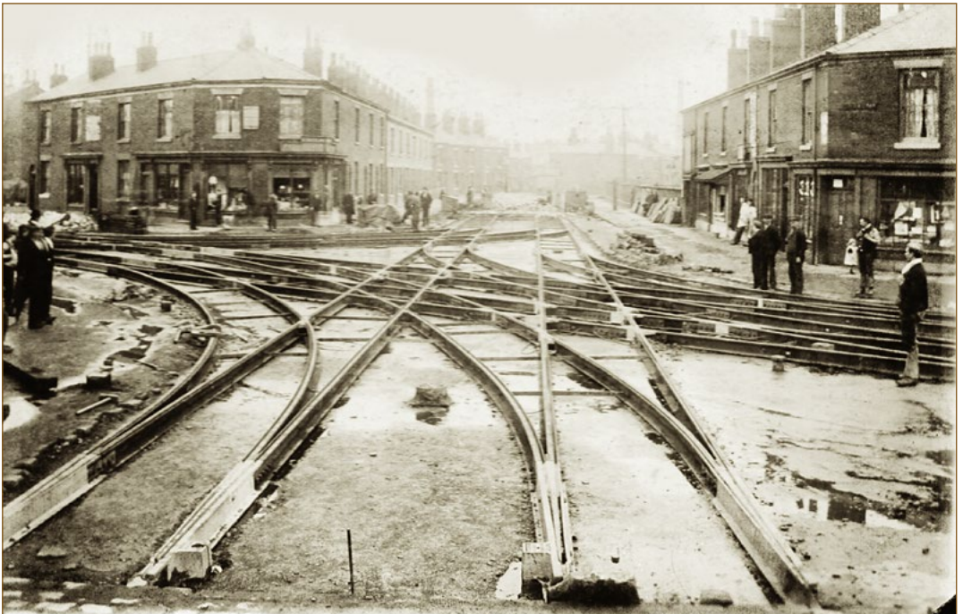
The junction of Long Causeway and Albert Road in Farnworth was a major piece of trackwork and, although not symmetrical, only one pair of tracks short of a grand union. Note the jim crow attached to the left hand curve in the upper picture – this was the implement used for manual bending of the rail to create curves or to modify and correct the geometry and gauge. Scenes like this would be familiar in towns throughout the country at this time. (66 Group)
