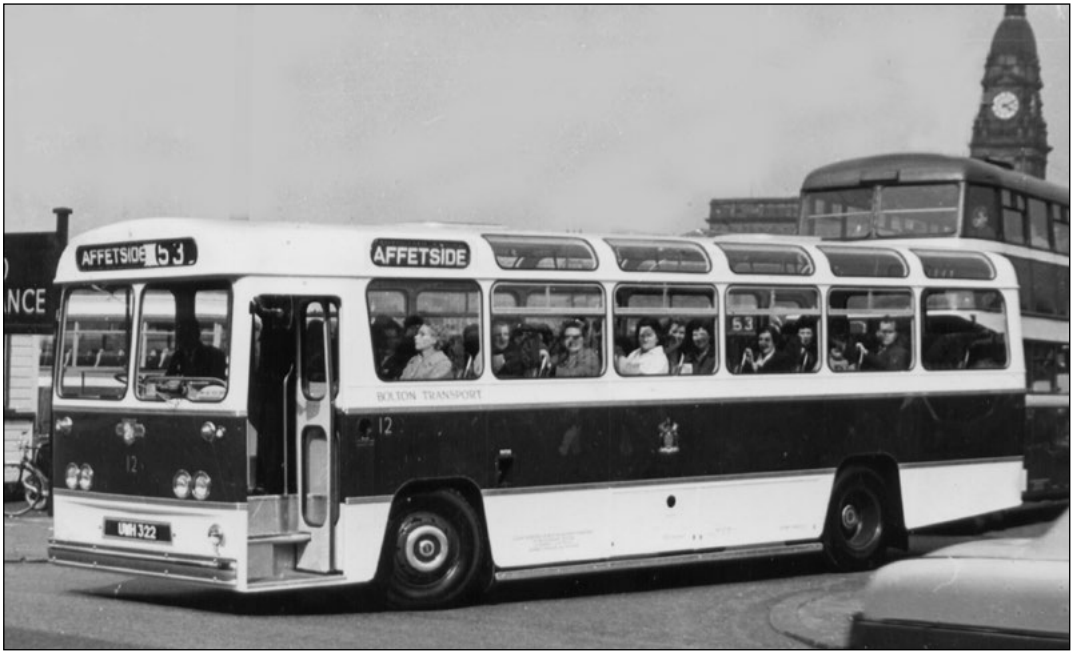
The first single-decker to be received since 1956 arrived in 1962 and was an East Lancashire Coachbuilders-bodied Leyland Leopard L2 with fleet number 12. It had dual-purpose high-back seating for 41 passengers together with curved glass cantrailis. It is shown above on more mundane duties leaving Moor Lane Bus Station for Affettside, and followed by a Leyland PD2/4 still in the maroon-and-three-cream-bands livery which now looks very dated by comparison with the Leopard. In the lower view at the other terminus the era of renovation and upgrading of the old cottages has clearly begun. ( BD, STA courtesy BCVM ).
