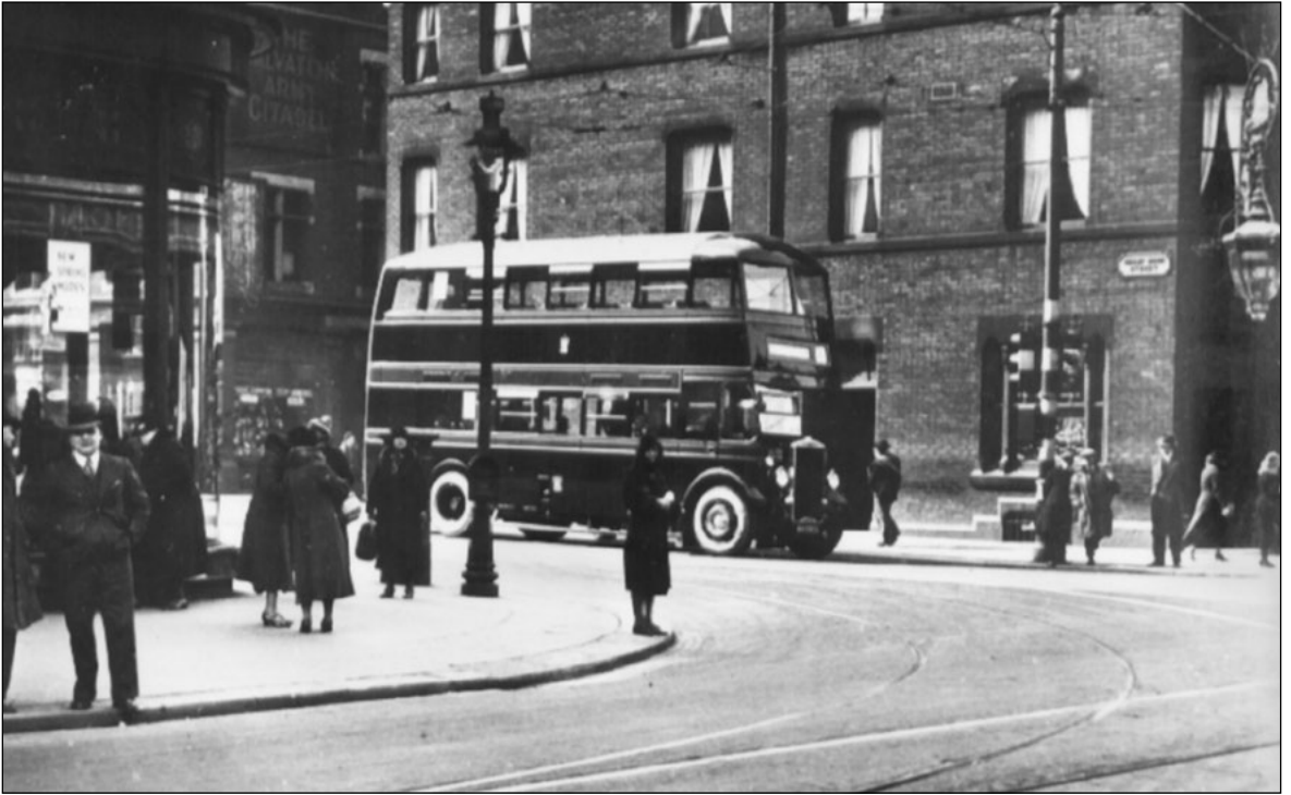
Taken in the summer of 1934, at the junction of Great Moor Street and Bradshawgate, the above picture shows Bolton No. 83, one of ten Bromilow & Edwards-bodied TD3s delivered that year, leaving for Brightmet and Bury, the trams having ceased the previous January. Note the revised frontal treatment; the 'piano-front' seen on pages 54/5 has given way to a smoother, unbroken outline. Number 83 was to be rebodied by Northern Coachbuilders soon after the war ended. (66 Group)
