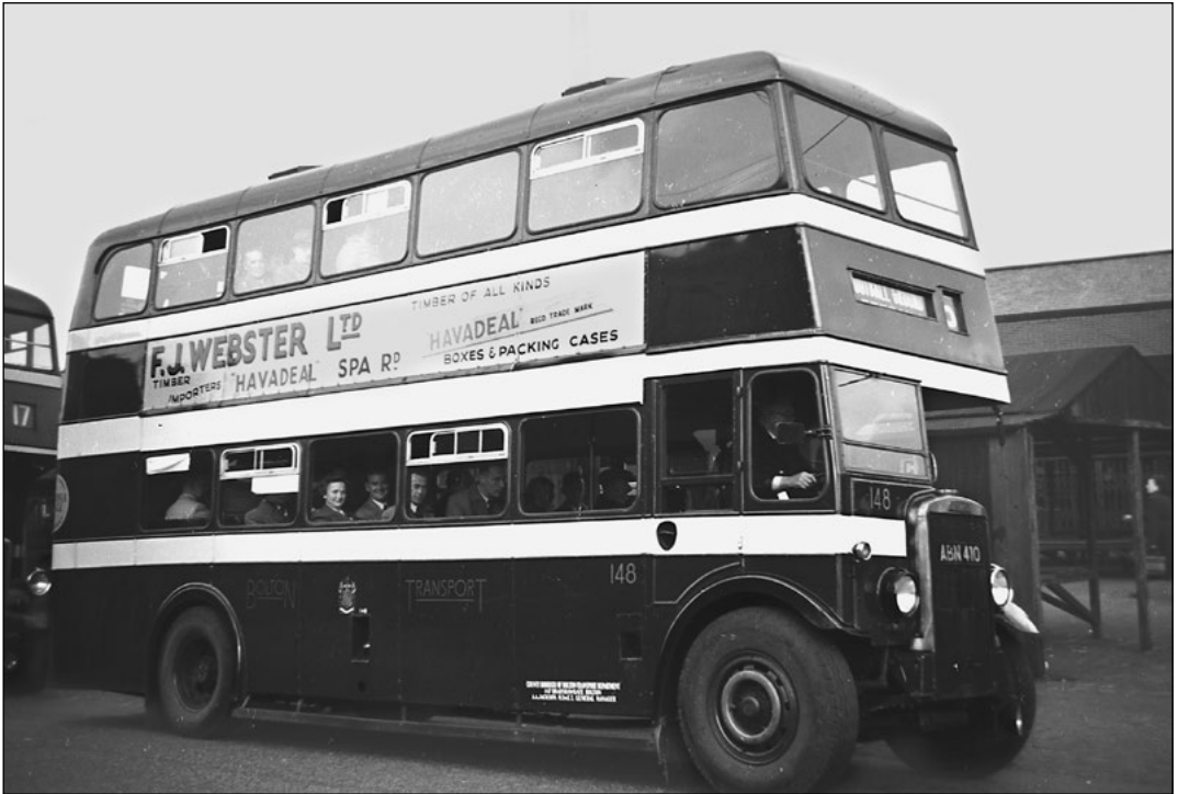
This view taken in October 1953 shows 1938 Leyland TD5c No.148 looking very smart having been rebodied with the 1945 'Relaxed Utility' Northern Coachbuilders body from No. 85. By this time the body had been the subject of rebuilding, including the provision of flush mounted perimeter glazing as can be seen. (AEJ)
