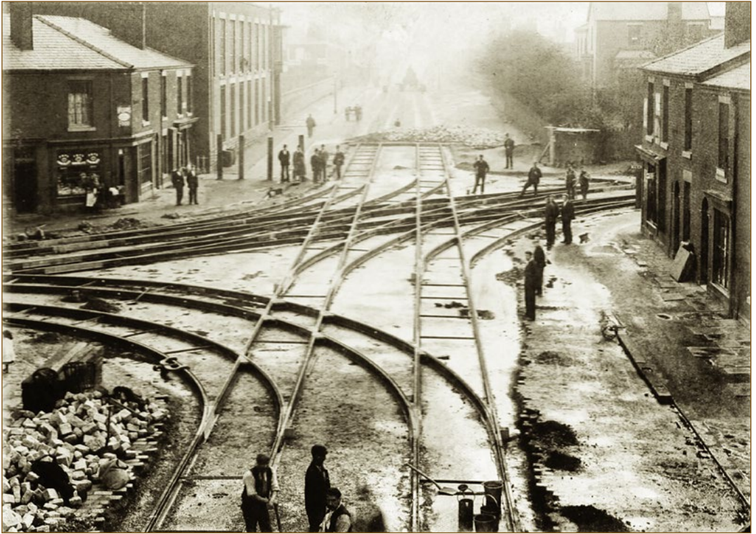
The junction of Long Causeway and Albert Road in Farnworth was a major piece of trackwork and, although not symmetrical, only one pair of tracks short of a grand union. Note the jim crow attached to the left hand curve in the upper picture – this was the implement used for manual bending of the rail to create curves or to modify and correct the geometry and gauge. Scenes like this would be familiar in towns throughout the country at this time. (66 Group)
