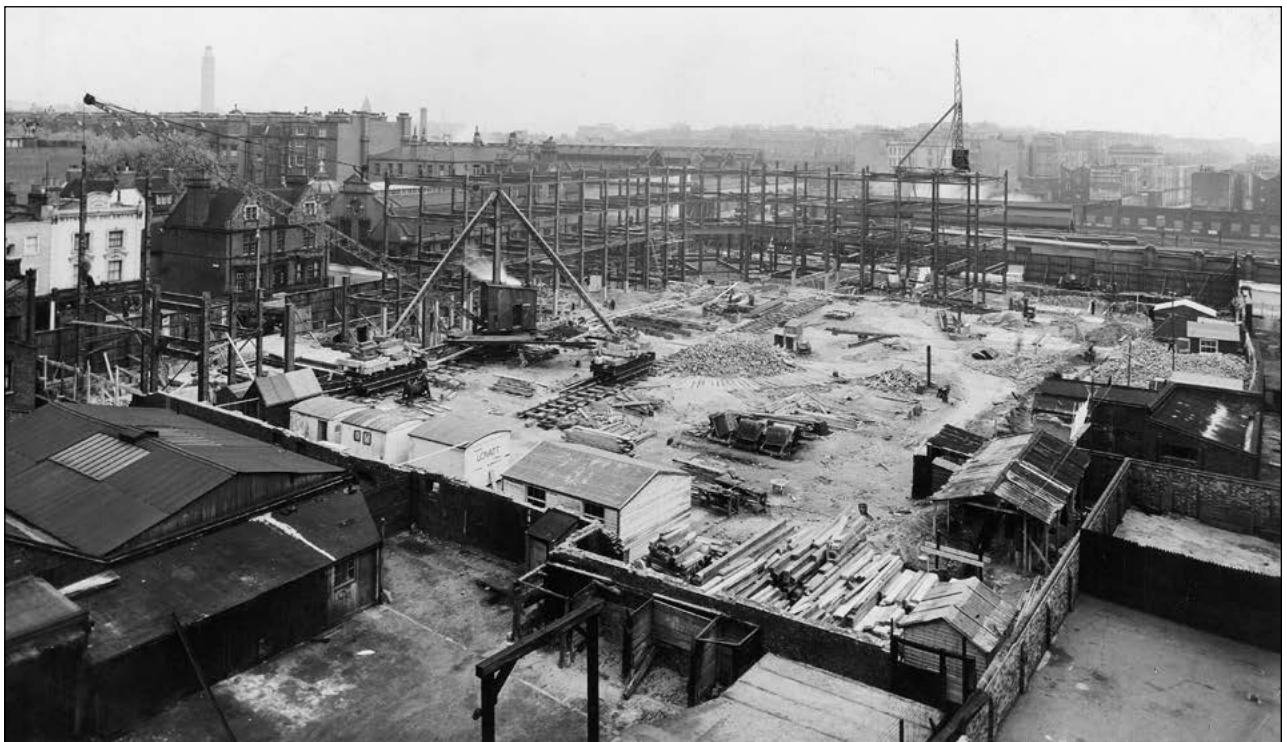
Almost four months since the press report shown in the previous illustration, and building work has started on the "super coach station". This is how it looked on 20th May 1931. (LCCc)
