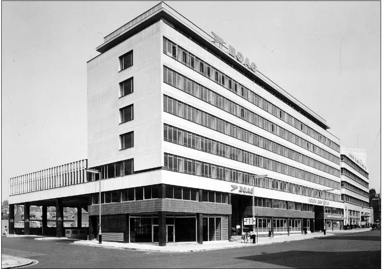
The impressive 1966 extension to the Buckingham Palace Road wing. Thereafter the coach entrance was from Semley Place beneath the single-storey extension (Fox Photos/LCCc)
