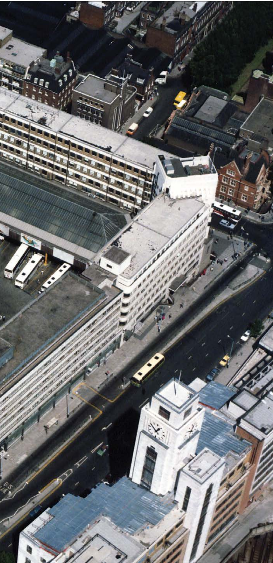
An aerial view of Victoria Coach Station from a later period showing how well the new extension matched the original building (more than 30 years its senior) and the new canopies over bays 15-22. BOAC Airways Terminal is seen in the bottom right hand corner in front of the (hidden) railway tracks from Victoria. (Peter Scammell collection)
