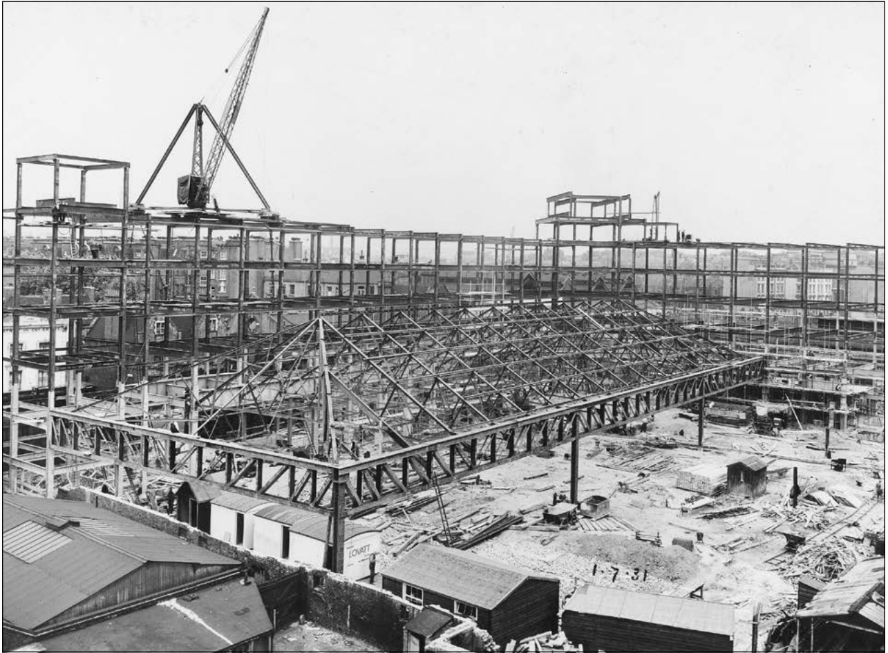
The coach station taking shape; this picture shows the state of progress on 1st July 1931. (LCCc)
