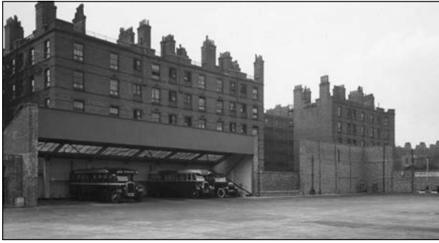
Three pictures showing alterations to the western wall of Victoria Coach Station (backing onto Peabody Buildings). The first, taken in 1932 soon after the official opening of the coach station, shows the small undercover arrivals or service area almost as originally planned; the second shows how much provision had been made for arriving passengers, including an adequate area for meeting and greeting; and the third shows the original service area having been converted into inspectors' offices – the arrivals platform remains unchanged, but obvious advantage has been taken of advertising potential. (LCCc)
