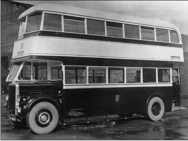
Upper. Although delivered a year later than 91, English Electric's rather antiquated 6-bay body makes Leyland TD4 number 108 (BU 8863) look the older of the pair. It was also withdrawn in 1948 but went for scrap. (STA)
