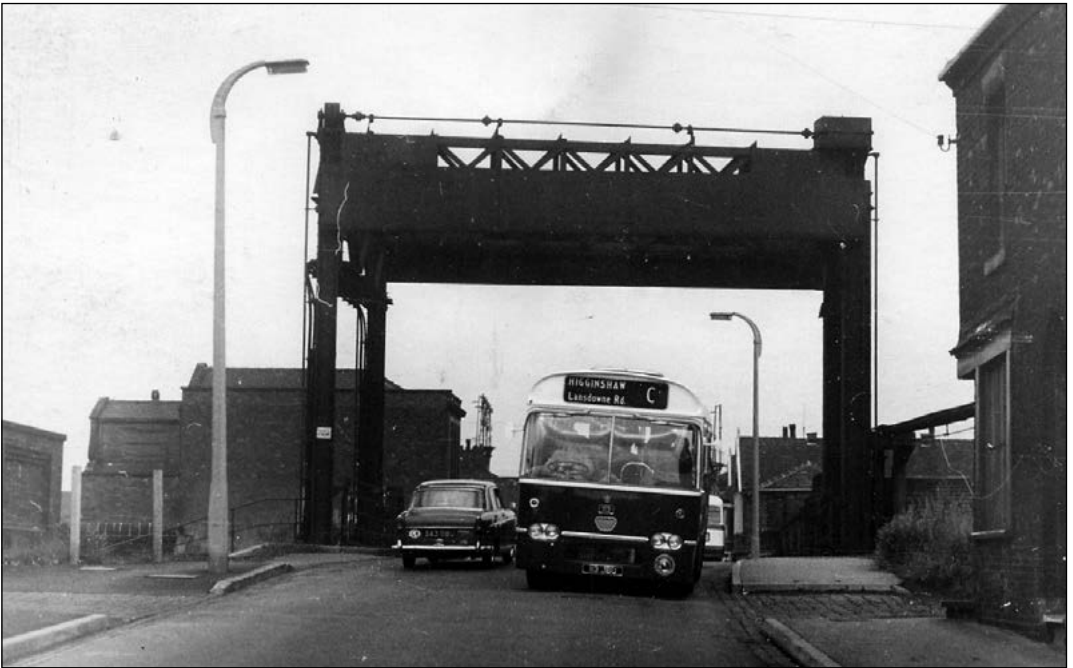
Upper. Between Shaw and Newhey, Jubilee Bridge crosses what was once the Oldham to Rochdale railway line, soon to become part of the Manchester Metrolink network. A notorious accident spot, Atlantean number 145 (GBU 145D) negotiates it on its way to Manchester. (JJH)
