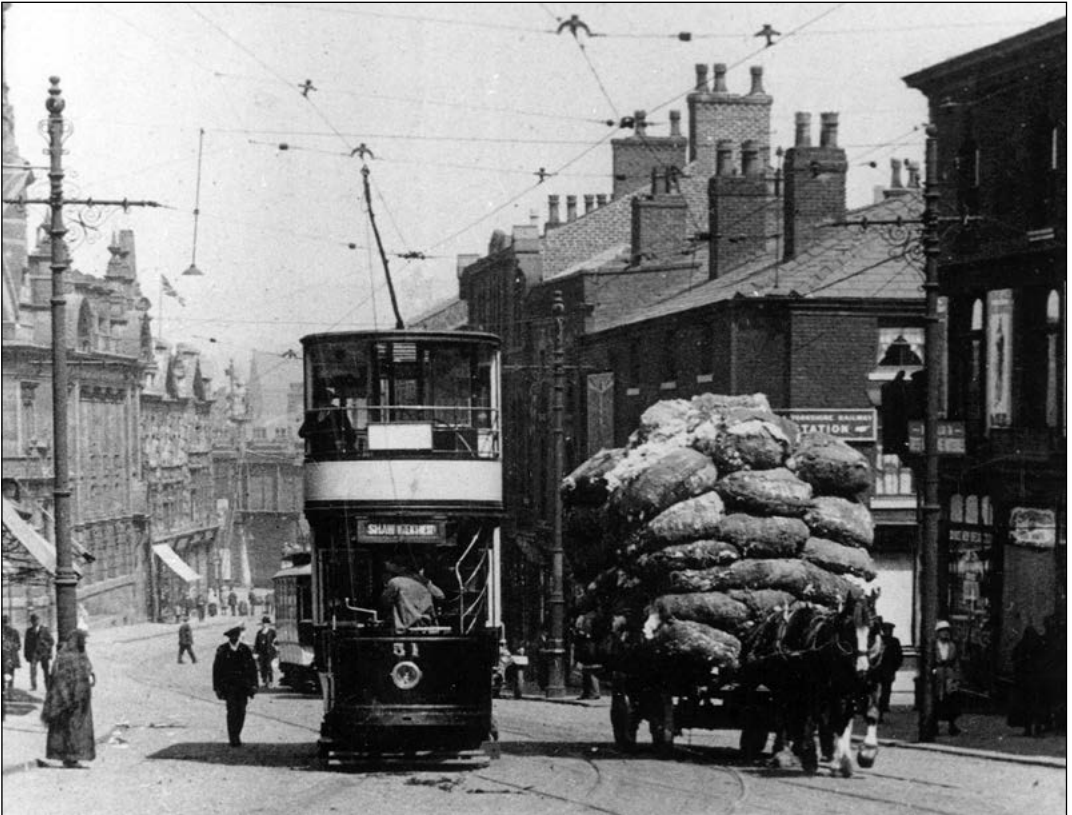
Tram number 31, new in 1902, had already received a top cover when it was photographed some ten years later at Rhodes Bank on its way to Shaw. The tram has just come down Yorkshire Street and Mumps railway bridge can be seen in the background. In this scene, typical of the times, a cart horse labours up the hill in the opposite direction pulling a load of cotton bales. (STA)
