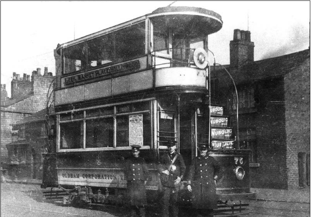
The new depot and workshops at Hollinwood were opened in 1910 when the expanding fleet outgrew the Wallshaw Street site. In the upper view tram number 36, now fitted with a Bellamy-type top cover, stands outside the ornate front of the depot about 1913 before leaving for Lees. In the lower picture, taken about the same time, the crew of number 75, another Bellamy car, pose for the photographer at the same point but looking back towards Manchester. (both STA)
