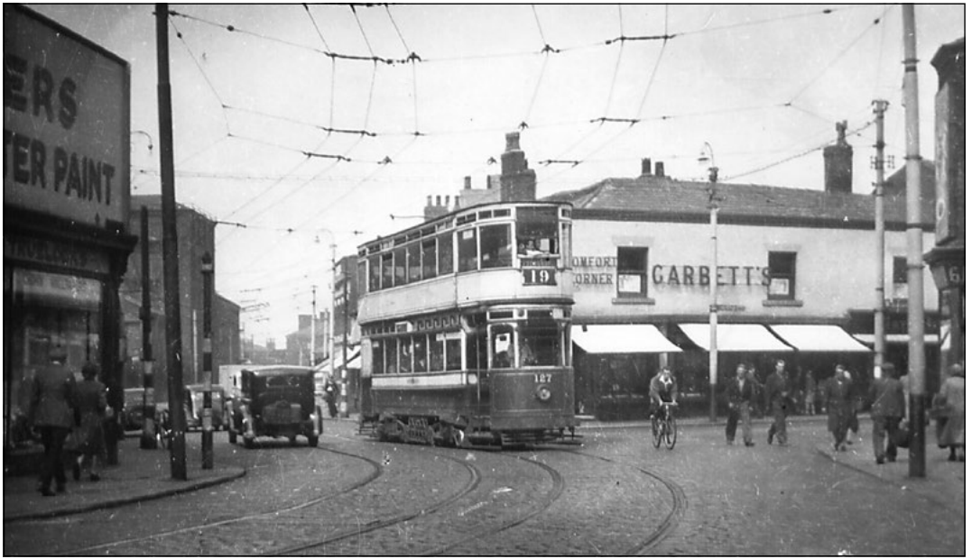
The system of keeping tram and trolleybus overhead separate, used extensively in the centre of Manchester, is clearly shown in this view, above, actually taken in the centre of Hyde. (JSKC)
