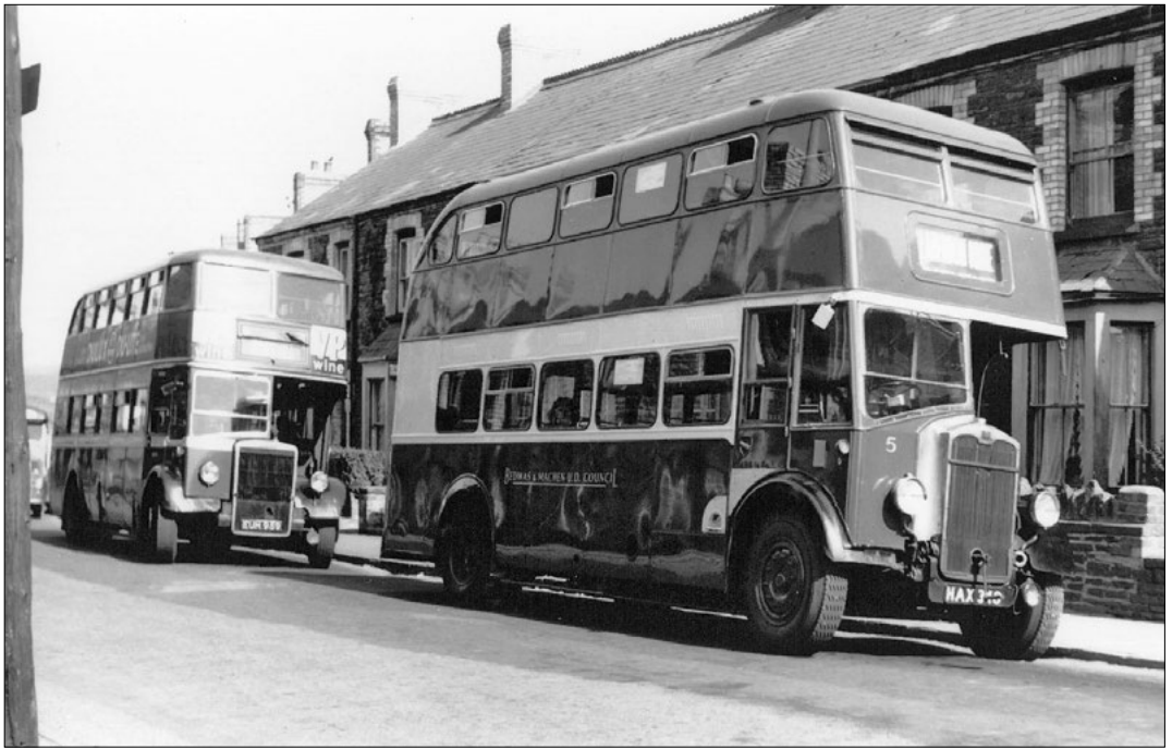
In 1954 HAX 340 was refitted with conventional rubber mounted windows and is seen here in 1958 in its later state, in Caerphilly.
