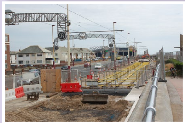
A new platform stop nearing completion at Norbreck in August, and track laying on the stretch leading to the Starr Gate loop, with the new depot just visible in the distance. (Harry Postlethwaite; John A Senior)
