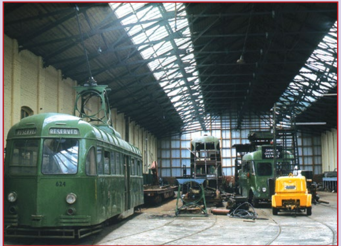
Blundell Street, now partitioned off and partially used by the permanent way department. Brush car 624 has become the engineering car whilst behind is an underframe from a scrap victim. To the right of the sorry-looking Balloon is one of the former Manchester Guy tower wagons. (G Lumb)
