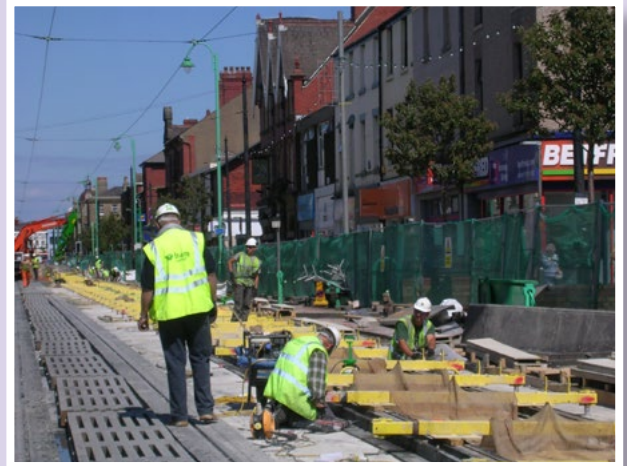
Relaying the tracks in Fleetwood during the Spring of 2010. (Harry Postlethwaite)
