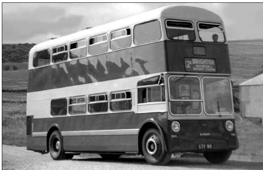
Leyland's Lowloader on demonstration with Southdown in 1954. It had a rear entrance with a turbocharged Leyland O.350 engine fitted transversely also at the rear. (Southdown Enthusiasts Club)
