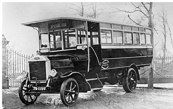
TB 1159 with its new body - started by BCLE it was almost finished when the firm became insolvent; LUT took it and finished the work.
