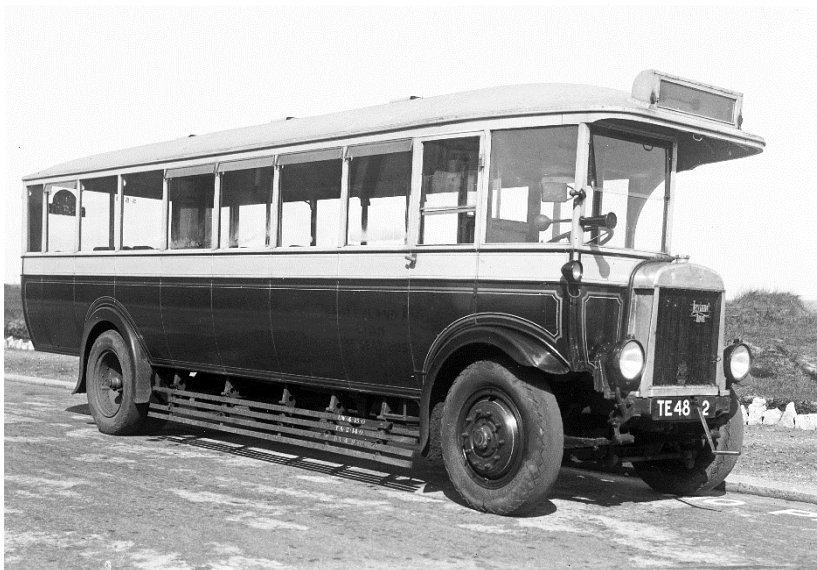
Leyland demonstrator TE 4812 was a PLSC equipped with the new engine and transmission that was to be used in the forthcoming LT1 Lion. LUT had it on loan and subsequently bought 73 of the new Lion model.
