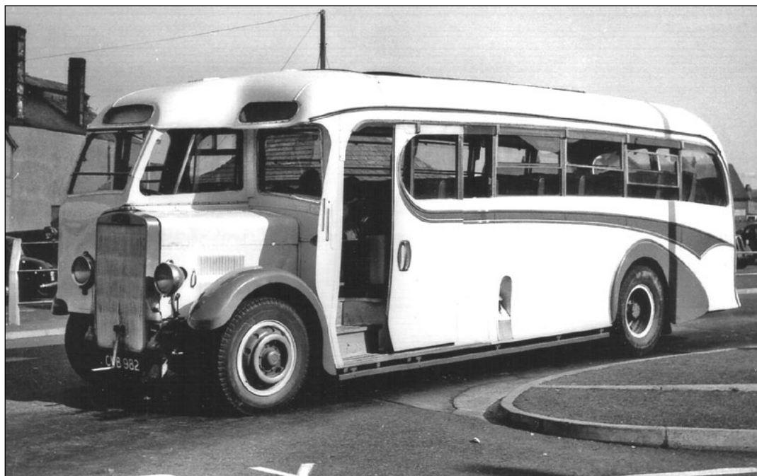
CWB 982 was originally a double-decker supplied to Sheffield Corporation in 1936. After the war the Leyland TD4c Titan was acquired by a dealer who scrapped its first body and replaced it with a 33-seat coach unit by Burlingham. Caelloi Motors of Pwllheli bought it in June 1958 and kept it in service until February 1961. ( Roy Marshall via the Omnibus Society )
