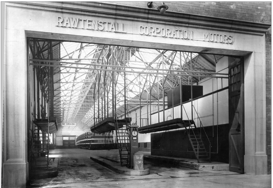
A view of the entrance to the new bus depot at the Bacup end showing the gantries for vehicle washing. Also visible is the name over the door – Rawtenstall Corporation Motors – still to be seen in 2007. (RT)
