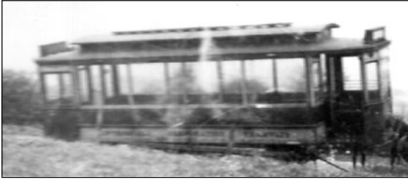
Single-deck No. 23 from the batch 19-24 survived as a shed for many years until purchased as a restoration project. Sadly, although it still exists, the necessary resources in terms of manpower and finance have not been available to allow the project to be completed. It had been hoped that the rebuilt car, on a replacement standard gauge truck, might one day operate in Manchester's Heaton Park with other restored electric trams. (RLIB)
