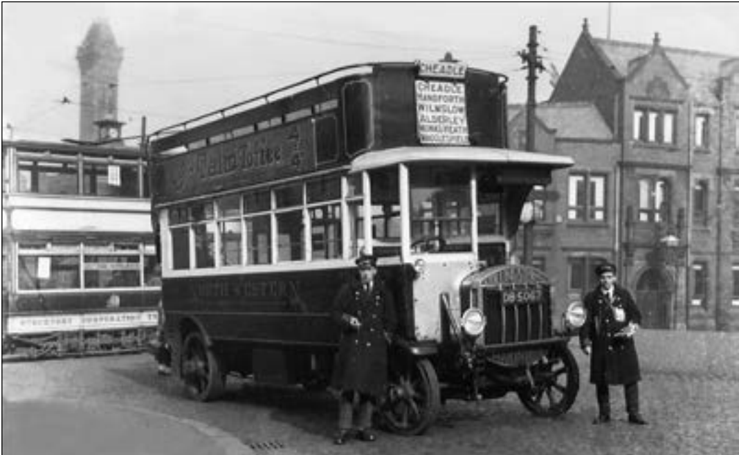
One of North Western's striking Brush-bodied Tilling Stevens petrol-electric buses is seen in Mersey Square soon after delivery in 1925. It is operating on the former British route to Cheadle. The petrol engine drove a dynamo which produced the electricity for an electric motor which powered the vehicle. Remarkably, one of these fascinating vehicles survives, fully restored, in the Museum of Transport in Boyle Street, Manchester. After withdrawal many passed to fairground showmen who were able to use the dynamo's output to power their attractions. The scene below also dates from the mid-1920s and shows a selection of buses undergoing maintenance and repair in North Western's Charles Street workshops. (STA both)
