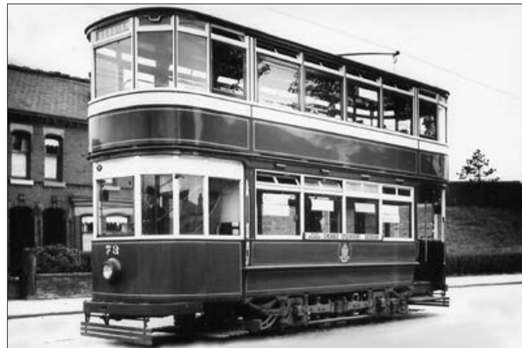
In 1939, just before the arrival of the Leyland TD7s below, the tramcar livery for the totally enclosed cars was modified to bring it in line with the buses, but there was later a small modification to the rocker panels (below the waist where the crest can be seen) which reverted to white. The route board is seen below. (MMC; JAS; STA)
