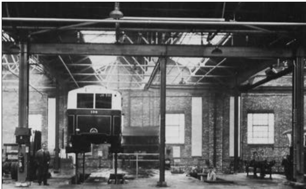
The steady increase in numbers of buses in the fleet – 46 by 1929 – necessitated extending the Mersey Square depot to provide accommodation and servicing facilities. Here one of the AEC Reliances stands on the hydraulic lift whilst awaiting routine attention. Note the chassis to the left. (MM courtesy Chris Heaps)
