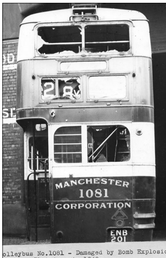
Reference is made in the text to the damage sustained by Leyland TTB4 No. 1081 on August 1940. Wartime photography was severely restricted, generally on the grounds of security, but these official views clearly show the damage sustained in what was described as a 'bomb explosion'. (GMTS)
