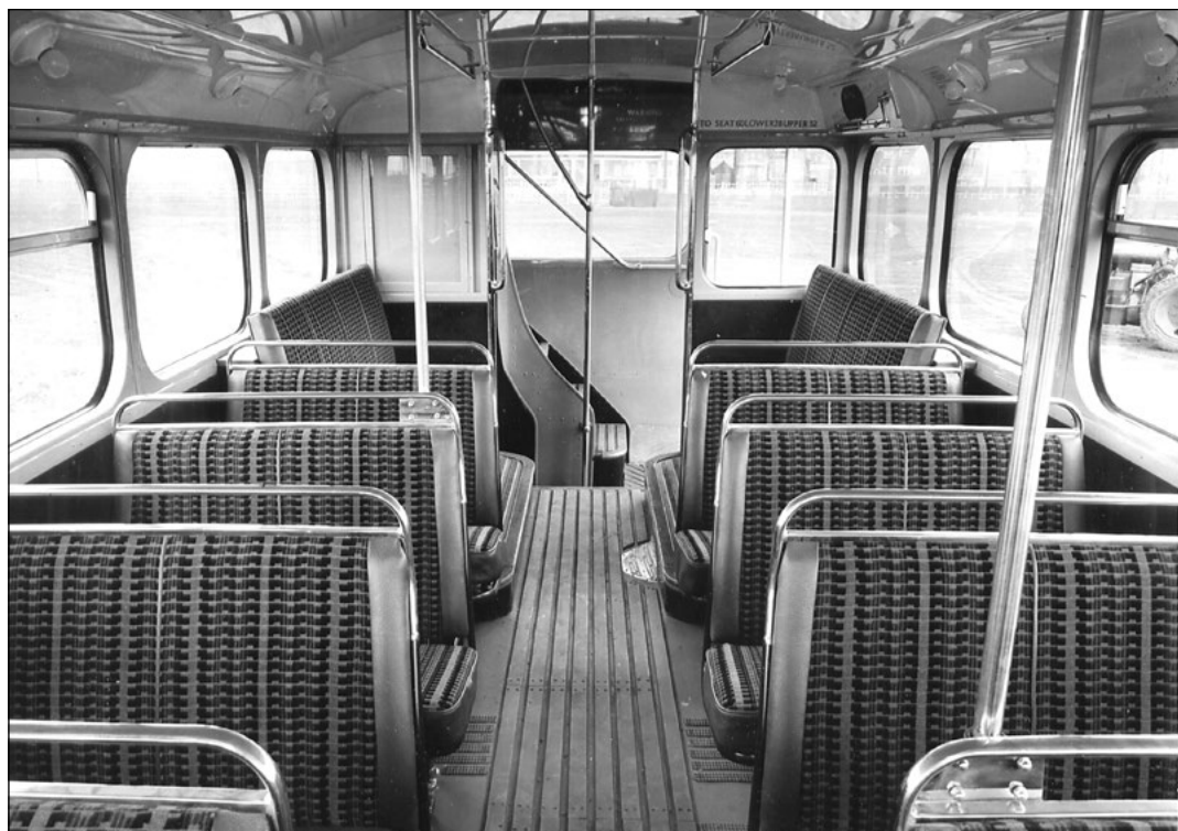
The interior views of the Burlington trolleybus bodies show attractive moquette seating in the lower saloon and brown Rexine-covered seats in the upper saloon, moquette not being considered appropriate in an environment where smoking was still customary. (GMTS)
